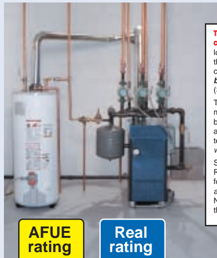
Conventional gas boiler and water heater.
